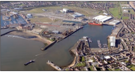
The new factory has 900m of quay with water depths of 8.5m. Pictured alongside is the Helix vessel MV Express.
